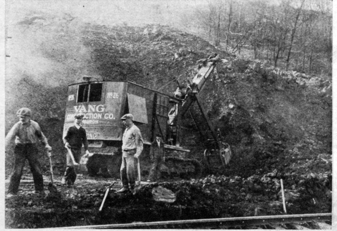
Left—Slide at Sta. 329 from Grade Above; Right—Koehring 1 1/2-Yd. Gasoline Shovel at Work on State Highway at Foot of Slide
